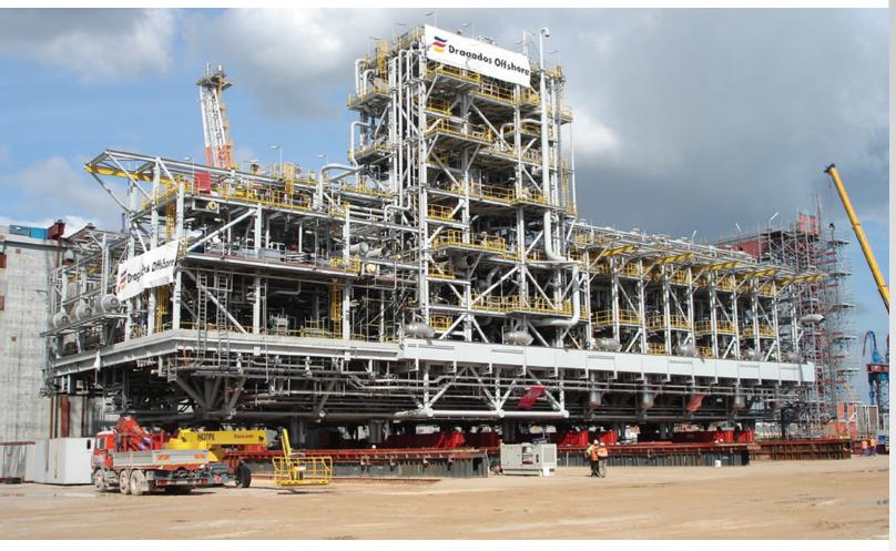
Construction of the world's first LNG regasifier, built with 90.000 m³ of cement and 30.000 ton of steel, required lifting and skidding solutions that could stand up to these extreme conditions. Enerpac HSK-Series skidding systems, in conjunction with HSL-Series heavy lifting strand jacks, provided the solution, which compensated for skidding on uneven ground, and lifting deck modules and equipment of up to 3000 ton.
