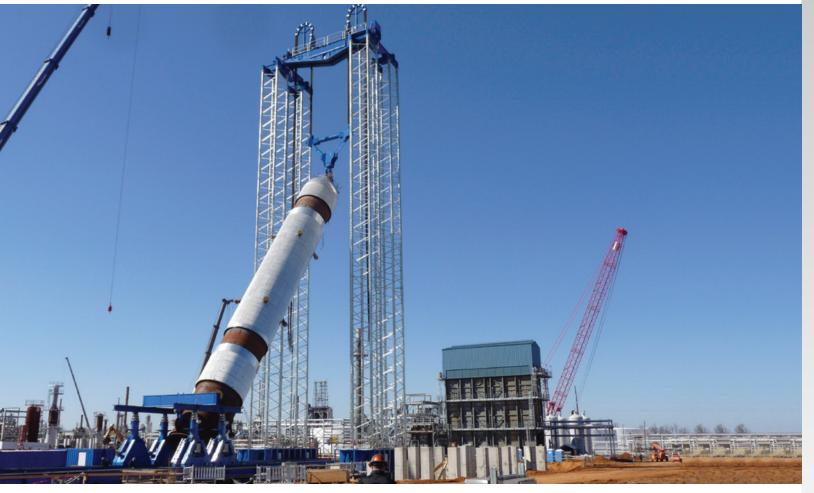
The Enerpac self-erecting tower combined strand jacking with hydraulic gantry and skidding technologies to form an integral, free-standing heavy lift and tailing solution. Transported in standard containers, automatic erection and takedown was completed at ground level, requiring only simple cranage to lift the header's beams prior to raising the tower. This provided a 1200 ton by 50 meter lifting solution that was quickly and safely set up in a 'live' environment at low cost.
