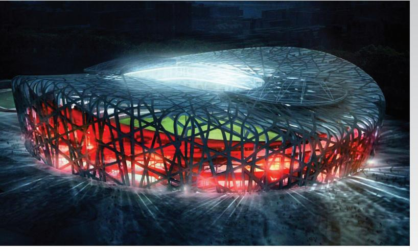
Beijing's National Stadium provided a spectacular venue throughout the 2008 Olympic Games. The steel roof lacked structural integrity during construction, requiring the use of temporary supporting works. After the last piece of the 45.000 ton roof structure was installed, it needed to be 'de-propped.' This delicate procedure was managed by Enerpac Synchronous Lifting Technology, allowing the structure to vertically relax downward into exact position with the removal of temporary works.
