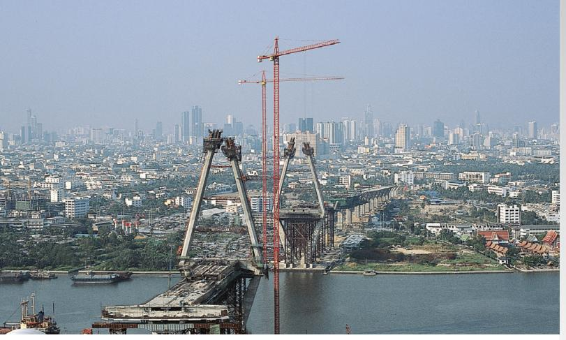
The industrial ring road was constructed to relieve traffic congestion in Bangkok's main industrial areas. This project was comprised of two 700 meter long, 172 meter high cable stayed bridges, and 13 kilometers of road. Enerpac designed and supplied hydraulic systems to launch and position the 1200 ton traveling formwork system to build the elevated approach road sections.
