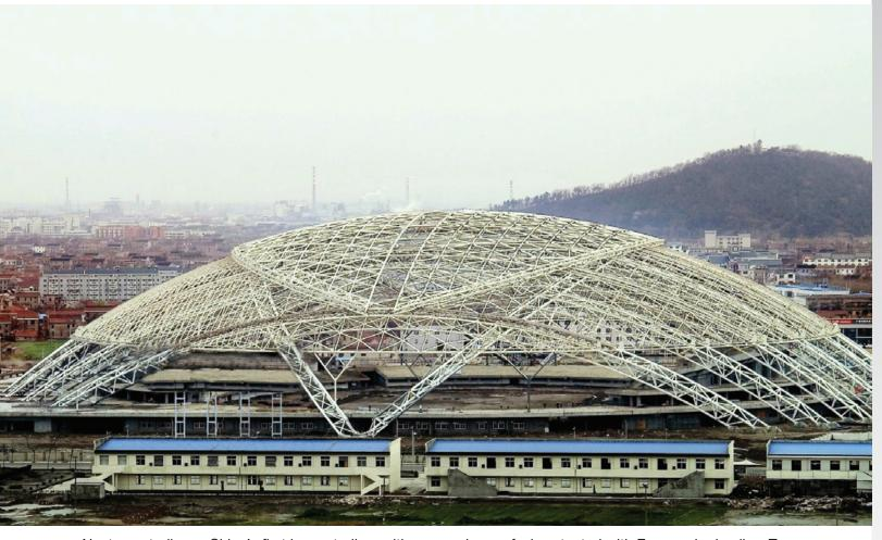
Nantong stadium - China's first large stadium with an opening roof - is actuated with Enerpac hydraulics. Two 1100 ton hemi-spherical roof shells, supported by hydraulic cylinders mounted on mechanical trolleys, are driven by hydraulic winches to open and close the roof structure 60 meters. Enerpac's solution synchronises the roof positions and manages the dynamic load conditions – all from a centralised location.
