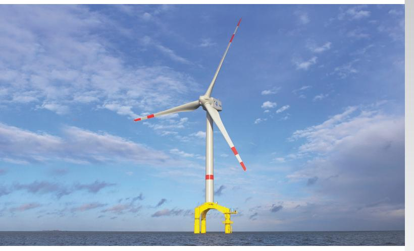
On the then first commercial offshore wind farm, wind turbines are installed with an Enerpac Synchronous Lifting System. The Enerpac system automatically adjusts and accurately positions the yoke on top of three deep pile foundations to provide a horizontal base. The turbine mast is then erected quickly and efficiently on the base.
