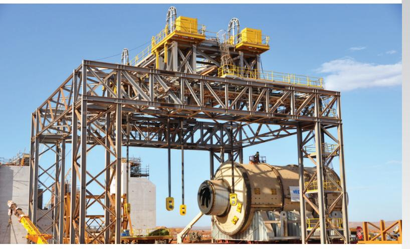
An Enerpac Strand Lift system was employed to construct Australia's largest ever magnetite mining and processing operation. With the HSL-series strand jack system, pairs of 800 ton iron ore mills and 1400 ton autogenous mills were lifted and then lowered onto their bearings 21 meters above the ground.
