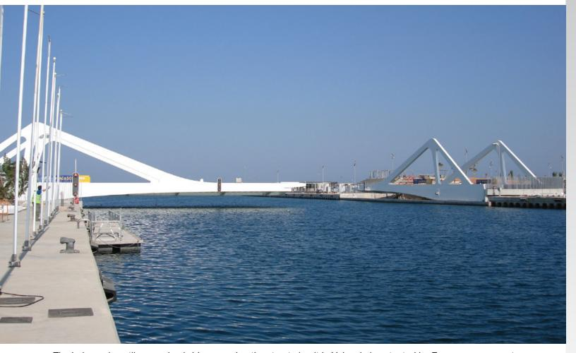
The balanced cantilever swing bridge crossing the street circuit in Valencia is actuated by Enerpac permanent hydraulic installation. Developed to allow yacht access in preparation for America's Cup, the bridge's design required a complex and failsafe digital hydraulic solution. Enerpac delivered actuation and a control system that successfully manages the 3200 ton counterbalance weight, spanning 99 meters, and operating 365 days per year.
