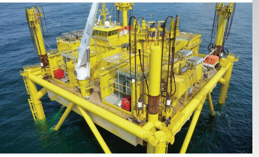
A salvage contractor's offshore platform installation was unstable and at risk. Enerpac presented the contractor with a fully engineered recovery solution to lift the platform to safety. Enerpac later supplied them with 16 strand jacks and 120 ton of fabricated structures, and soon the platform was lifted to its required elevation and secured.
