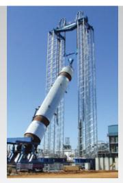
The Enerpac Self-Erecting Tower is a selferecting-tower-lift system that enables you to build a free standing gantry from ground level. The Self-Erecting Tower can be supplied in various capacities and heights and is built with standard modular components, enabling a flexible solution to future project demands.
