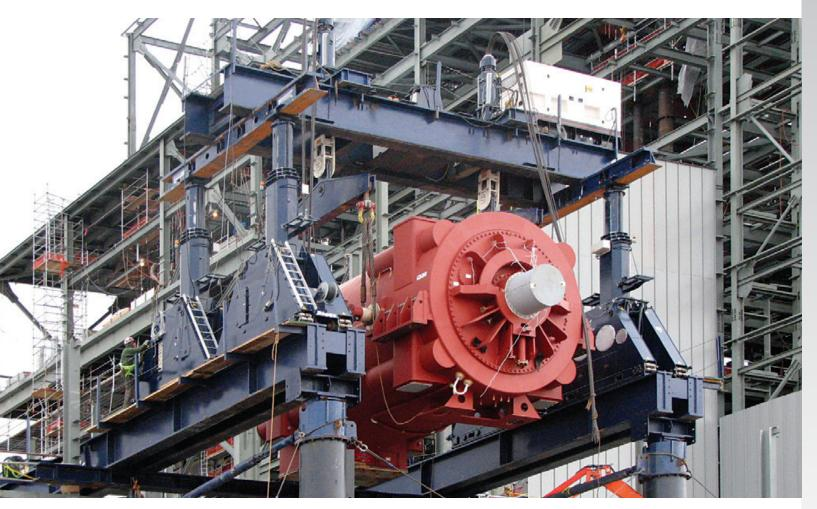
At a coal-fired power plant, HSL-Series Strand Jacks are used to lift power train turbine modules up to 250 ton, at a height of 14 meters. The self-propelled tank rollers of the SBL1100 hydraulic gantry traverse the turbine longitudinally, 70 meters along the elevated runway.
